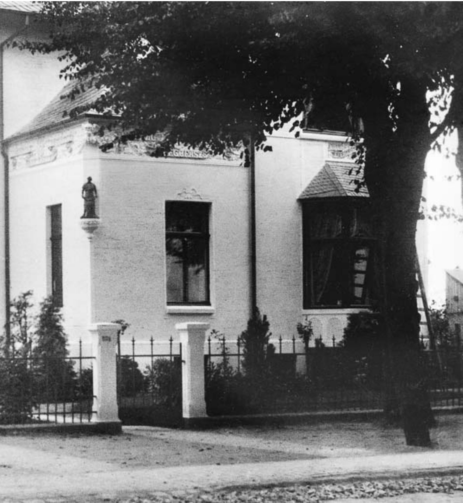
Around 1900 The "Old Factory" on Moislinger Allee, Lübeck.
